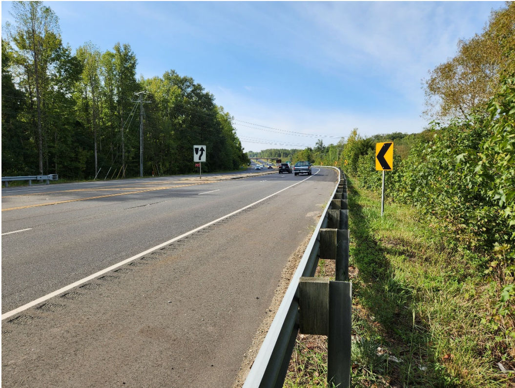
Photo #1: View to the southwest along Richmond Highway (US Route 1) and within the proposed CRPA encroachment for the proposed right-of-way improvements (September 21, 2023, by S. Gagnon, Bowman).
