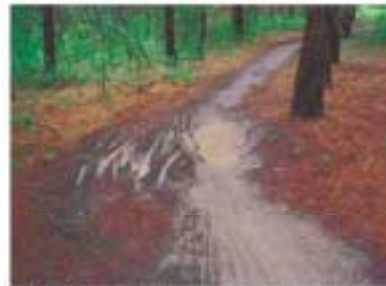
Problem: Trail creep. The low spot on a mountain side trail is gradually well. Having trail users to get around it. Careful removal of the down well roots as a threshold is necessary to avoid soil and vegetation of the trail.
