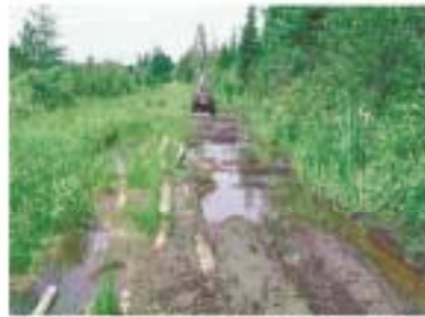
Problem: Compacted and displaced tread in lowest area makes the tread unsuitable. Attempting to drive the tread back into the same area unsuitably changing the hydrology of an adjacent wetland. Rerouting or closure of the trail is mandatory.
