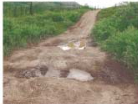
Problem: Trail splayed. If overuse occurs here and will not be corrected, it is inevitable that a trail will keep expanding until new options will be created. These problems are common in areas of erosion, with a lot of riding there is no real change. Rerouting or closure is the best solution. Where that is not possible, consider engineering using riding grade techniques and use of a low to deep water on the trail can help correct problems.
