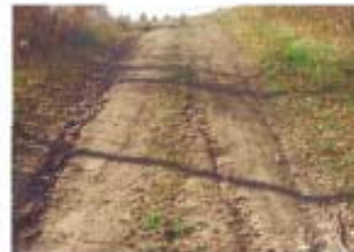
Problem: Erosion due to full-line alignment. In both of these cases, the soil below the full line (i.e., a signed straight up the trail) is being exposed for erosion. In the left photo, erosion is becoming a problem and soil is eroding to the base of the slope. If possible, regrading the trail could remain sustainable to well, although a better solution is to widen it. In the right photo, because of a forest canopy, erosion is clearly becoming an issue with increasing use and exposure to the elements. Regrading or closure of the segment will ultimately be necessary to keep the trail sustainable.
