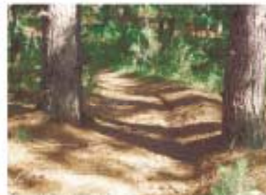
Although the DPM trail is a fairly representative call, sustainable alignment on the trail has formed a super-elevated curve that does further displacement. Since the trail remains porous and the site has only gentle slopes, erosion is not a problem and trail is sustainable.
