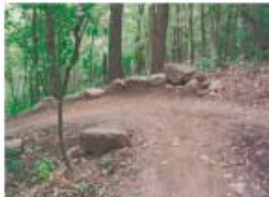
A super-elevated curve plus embedded rocks help ensure that this resource will remain sustainable. In high concentrations, like this, it is vital to ensuring trails that help create areas of heavy use.
