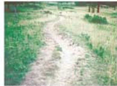
Problem: Soil rutting. With heavy use, trail creep can become a sustainability issue. If this is limited to an occasional rut, no major action is required. But if this problem persists over a significant distance, regrading or closure may be necessary.
