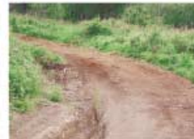
Problem: Severe, ongoing erosion on a roadless slope. Compacting the through characteristic of a site is a prescription for the kind of problem. The trail will have to be redesigned using riding grade techniques if it is to be sustainable. Otherwise, closure will ultimately be necessary as the problem gets worse.
