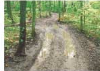
Problem: Compaction and displacement on a new-level site deepening the tread of this relatively new ATV trail. Visual search will find tread because it is the lowest point. Fixing the problem by improving drainage and perhaps hardening the tread through this section are possible solutions.
