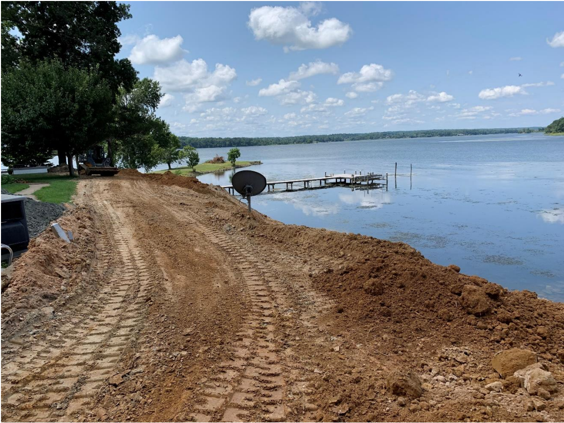
Photograph was taken facing south showing the western shore of Accokeek Creek after placement of fill and grading; August 4, 2021.
