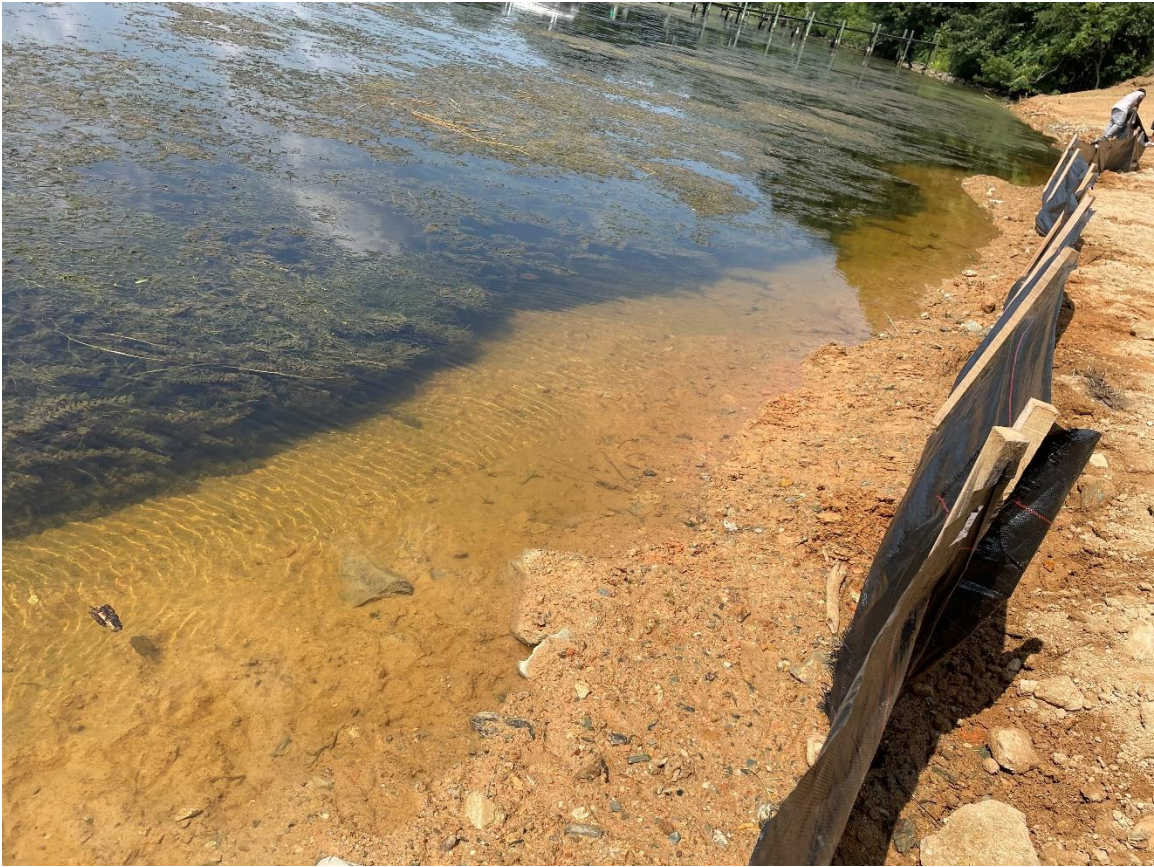
Photograph was taken facing north showing the installation of silt fence August 9, 2021.
