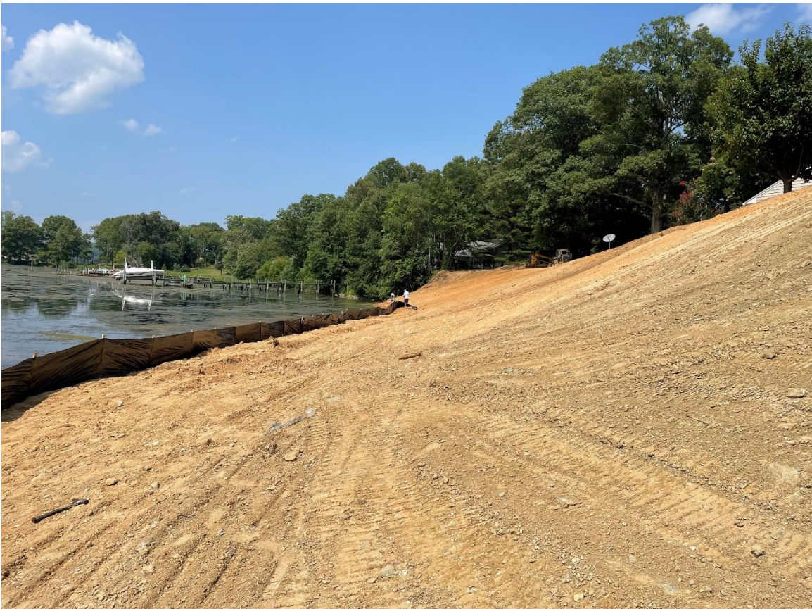
Photograph was taken facing north showing the filled and graded slope, and silt fence installation along the shoreline of Accokeek Creek; August 9, 2021.
