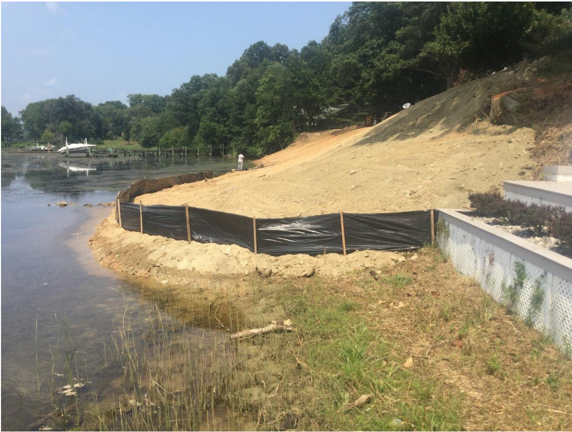
Photograph was taken facing north showing the filled and graded slope along the shore of Accokeek Creek, August, 4 2021.
