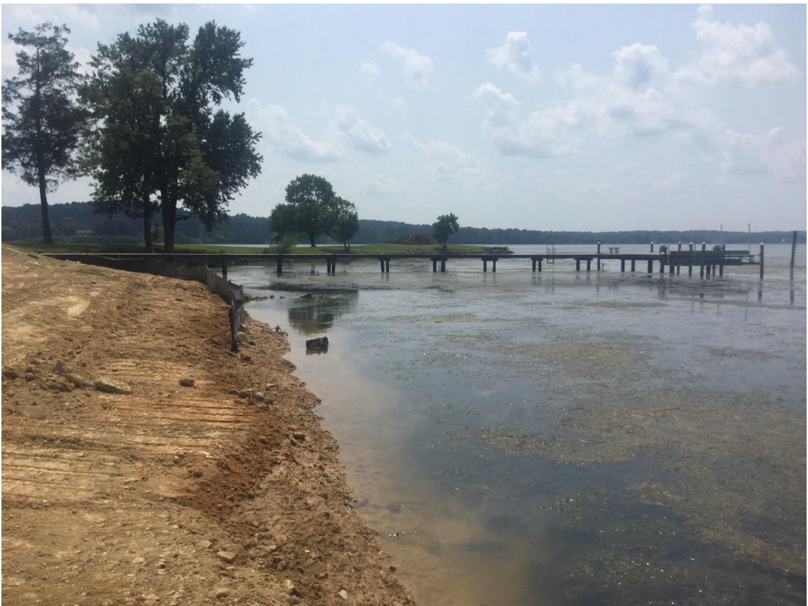
Photograph was taken facing south showing the installation of silt fence, August 9, 2021.
